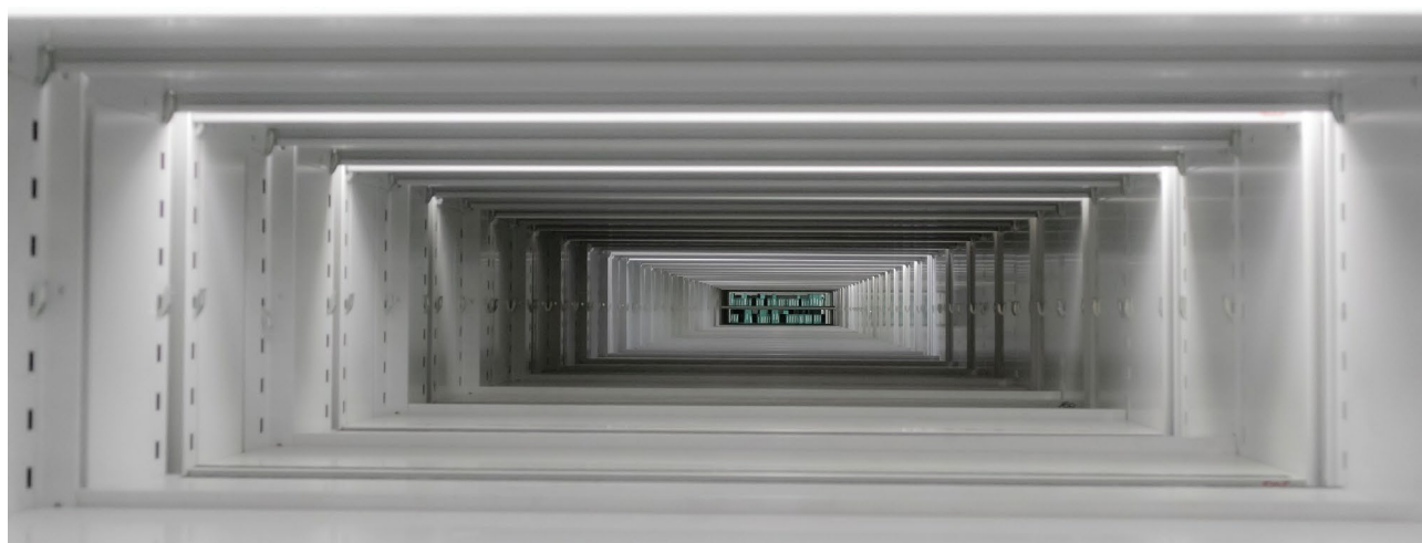
Figure 4. View through multiple sections of ORF empty vaults, showing some of the last cassettes to be migrated at the end of the shelves. © Photo by Christoph Bauer / ORF.
